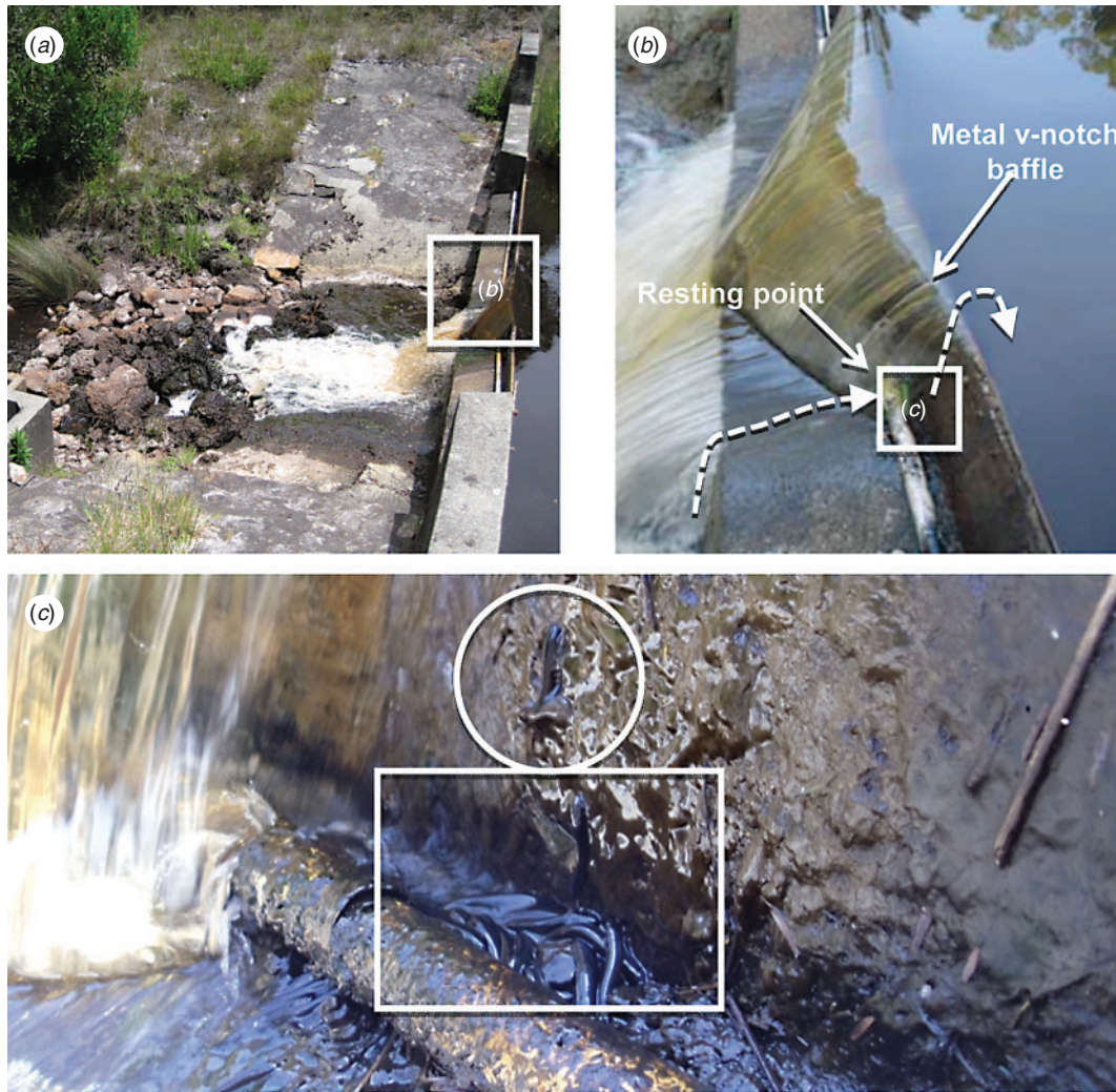
Fig. 1. The Goodga River weir and weir-skirt (a) over which juvenile Galaxias truttaceus were observed climbing and jumping (b). Boxes in (a) and (b) indicate areas enlarged in (b) and (c) respectively. Dashed arrows in (b) indicate ascension route. Box in (c) shows accumulation of Galaxias truttaceus below V-notch baffle and circle shows two G. truttaceus climbing the vertical baffle.
